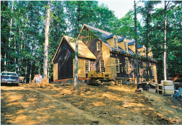
Under construction at last!
